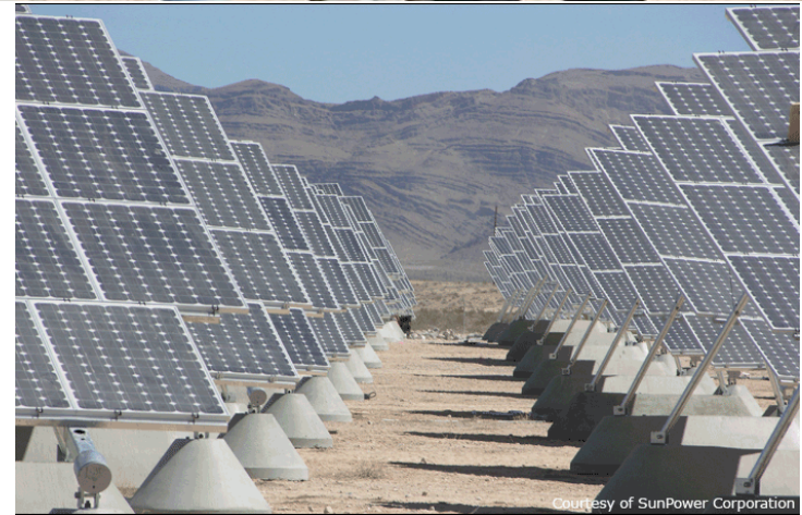
Courtesy of SunPower Corporation
