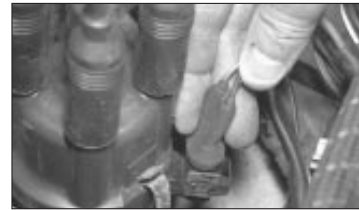
C Check that the LT lead connections are clean and secure.
