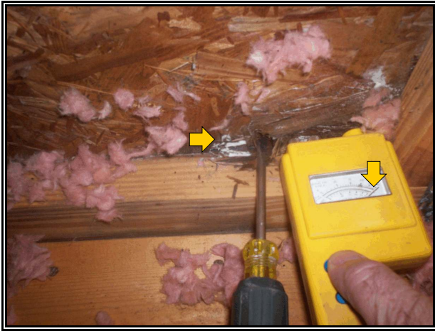
Photo 1- Wood decay and increased moisture at the base of the right gable end siding in the attic.
